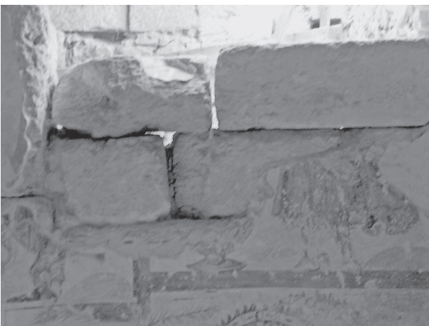
Fig. 4 - The slit in the wall from inside.
